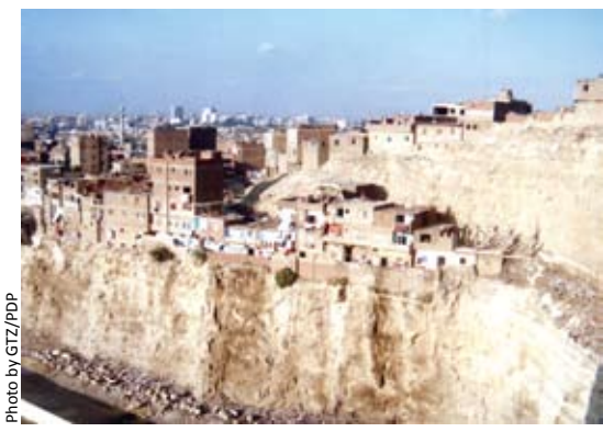
A typical unsafe area in Manshiet Nasser
