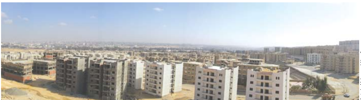
Alternative housing in el Doweiga, Manshiet Nasser
