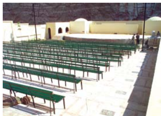
The upgraded cultural center and amphitheatre of Manshiet Nasser
