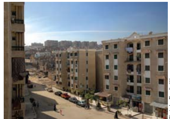
On-site redevelopment of el Doweiga, Manshiet Nasser
