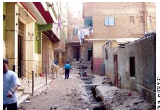
Infrastructure provision project in Manshiet Nasser
